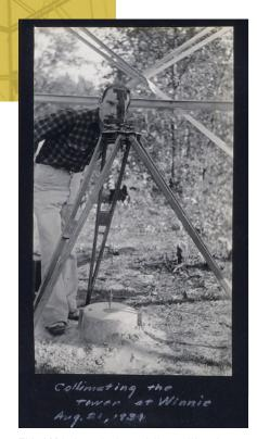
This 1931 photo depicts a fellow collimating a tower using an old K&E collimating instrument. The Indiana Bilby was collimated in the exact same manner but with a newer style instrument by Mike Fowler. Both the instrument mount on the top of the red (inner tower) and the light plate high above [74 feet] were aligned with the station on the ground.
