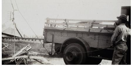
Manpower was specified and economical on the original tower crews. This ingenious method was designed to winch the heavy steel and other parts to the higher sections of the tower. Later designs of this method included a throttle within the rear fender of the haul truck so the rigger could control the speed of the payload on its way up.
