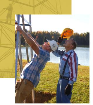
Joe Lindsay and Ulis Jones (retired USC&GS/NGS), both experienced tower builders and observers correct the alignment of the base. By sighting through the intersection of the diagonals (the midpoint of the horizontal ties) up through the tower, the foreman would direct the crew members to adjust the alignments of the inner (red) and outer (blue) towers.
