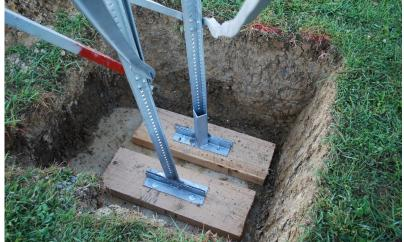
The alignment was accomplished through scooting the legs and anchors using steel pry bars. "Setting the base" was very important before the towers had reached heights of 74 or 87 feet and often more. The Indiana Bilby was set in concrete. In normal tower construction, the anchors were buried in dirt. In some cases, all that secured the anchors to terra firms were sand bags.
